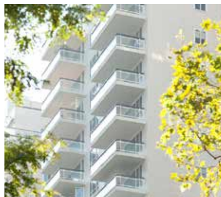
Manhattan House, 200 East 66th Street
